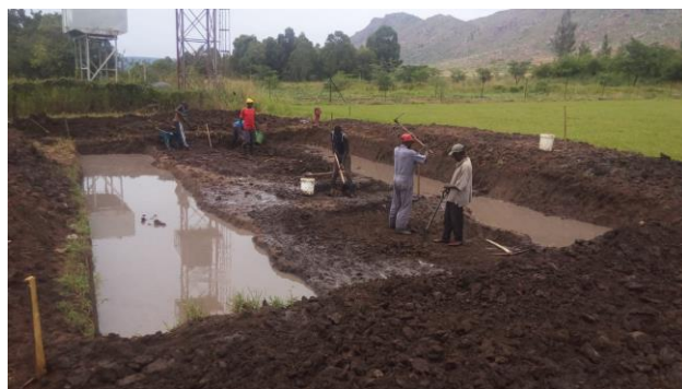
Photo 1: Construction of the Makini School fish pond
