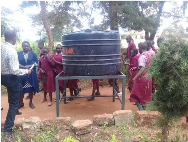
Photo 3: 500L water storage tank and stand for irrigation at Mutulani Primary
