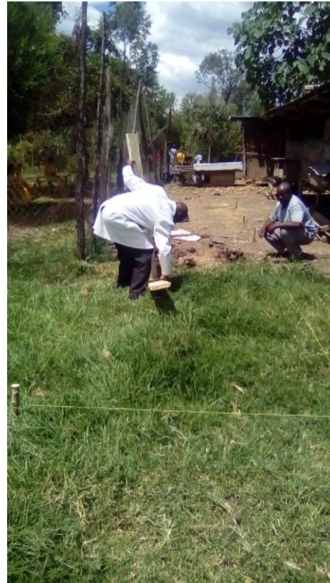
Photo 8: Construction of a poultry house at St. Theresa's Primary
